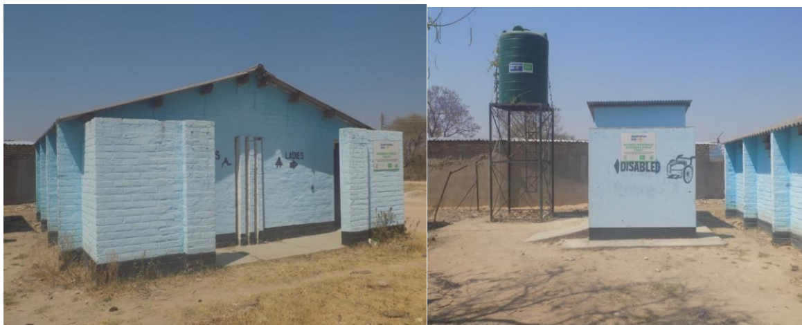
Whozhele Business Centre (Ward 11) public toilets (left) and disabled toilet (right) constructed in response to community priority and constructed by Sanyati RDC in partnership with Australian Aid
