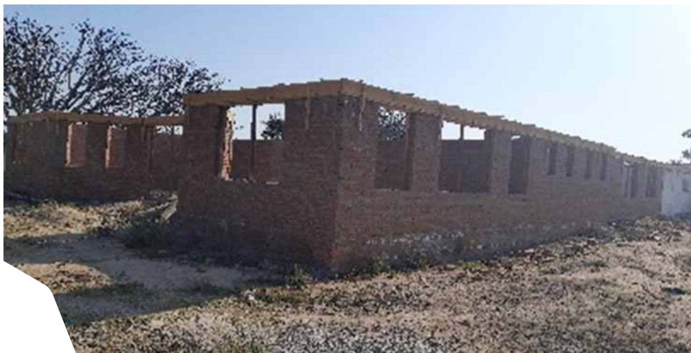
Ndakaziva Poly Clinic construction was begun after prioritization during the CBP process in Chikomba District
