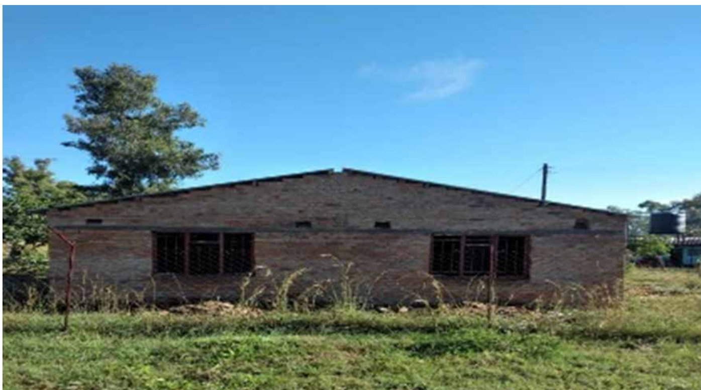
Gandami Mothers Shelter Constructed in Chikomba RDC after prioritization during the CBP Process
