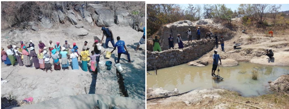
Women participating during the construction of dam in Mbudzi B ward 13, Mutoko district
