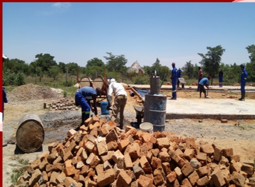
Digester Construction at Kanyandure Homestead in Mudzi District – Shinga Ward
