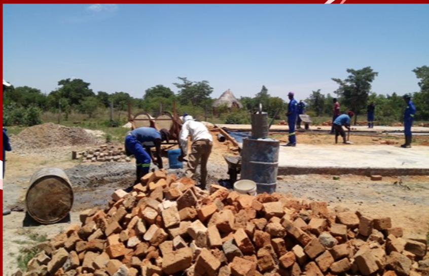
Digester Construction at Kanyandure Homestead in Mudzi District – Shinga Ward
