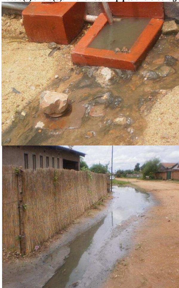
Plate 3(a) and 3(b): Broken sewer pipes and blockages
